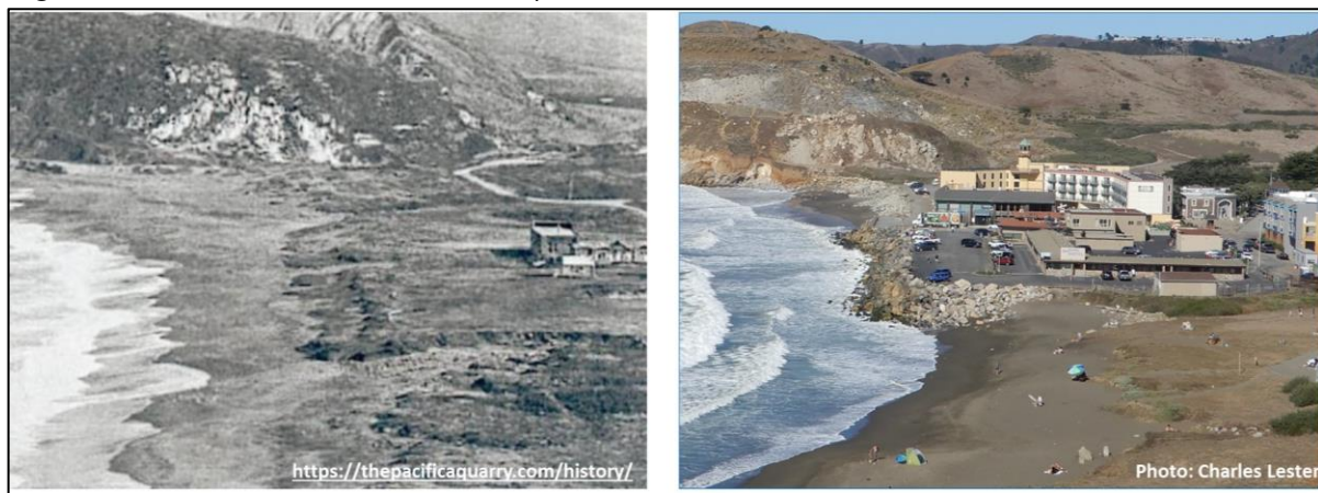
Figure 9. Loss of tidelands as development blocks shoreline recession, Pacifica.
