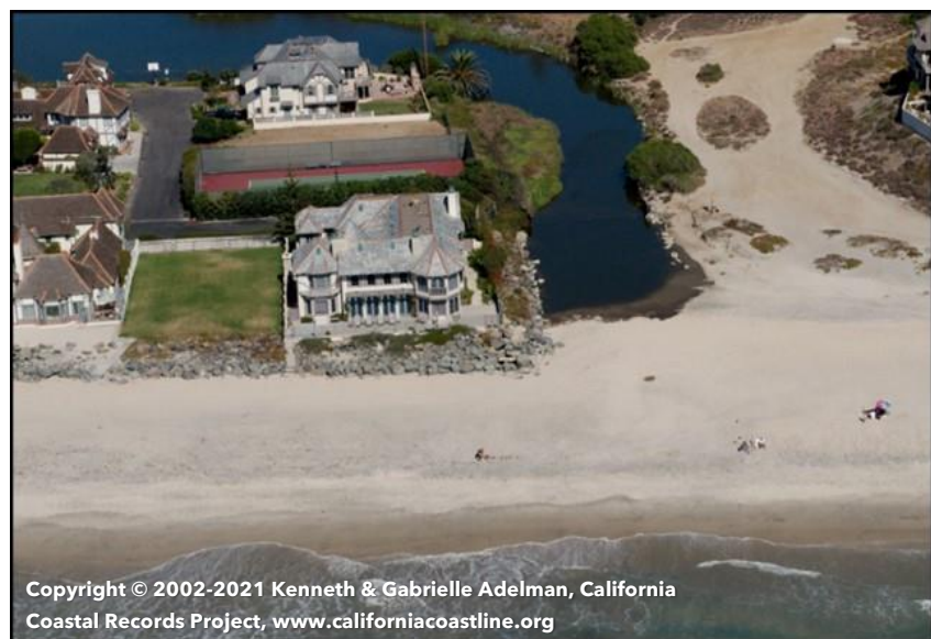
Figure 31. Buena Vista Lagoon Revetment Encroachment.
