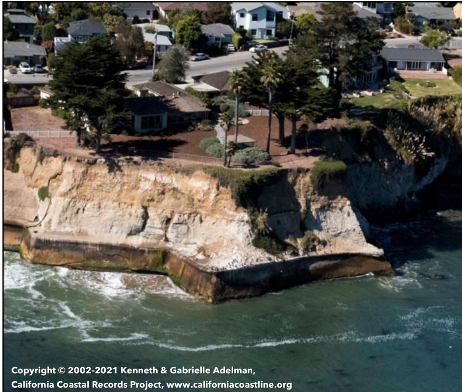
Figure 27. Shoreline Structure on Tidelands – Santa Cruz County.
