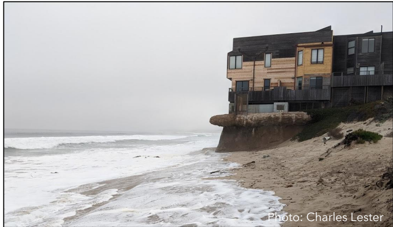
Figure 10. Ocean Harbor House at King Tide, Monterey.
